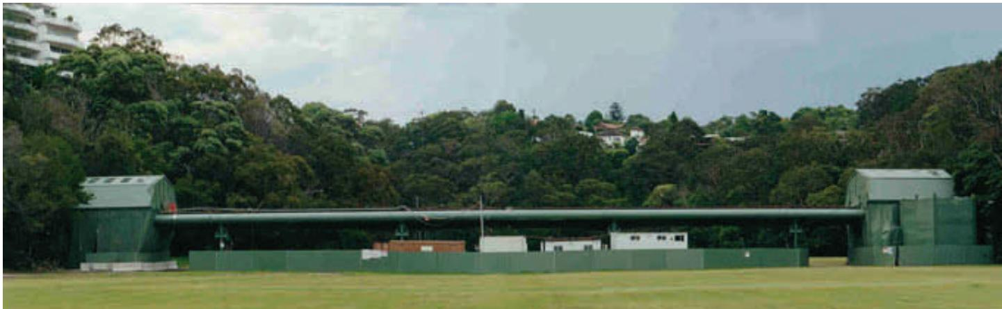
Acoustic Enclosures on both ends during internal repairs to the 80 m long reinforced concrete Sewer Aqueduct
